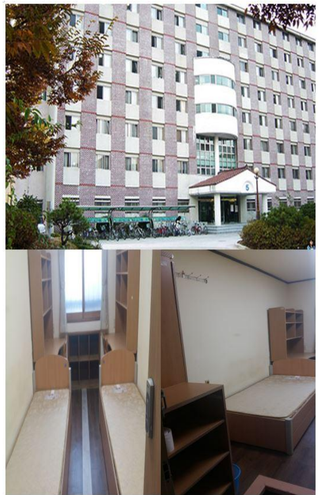
Building 5 (interior, exterior)
