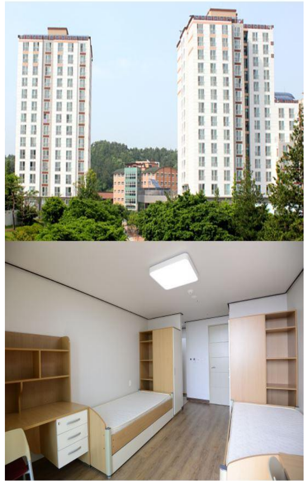
Building 10 & 11 (interior, exterior)
